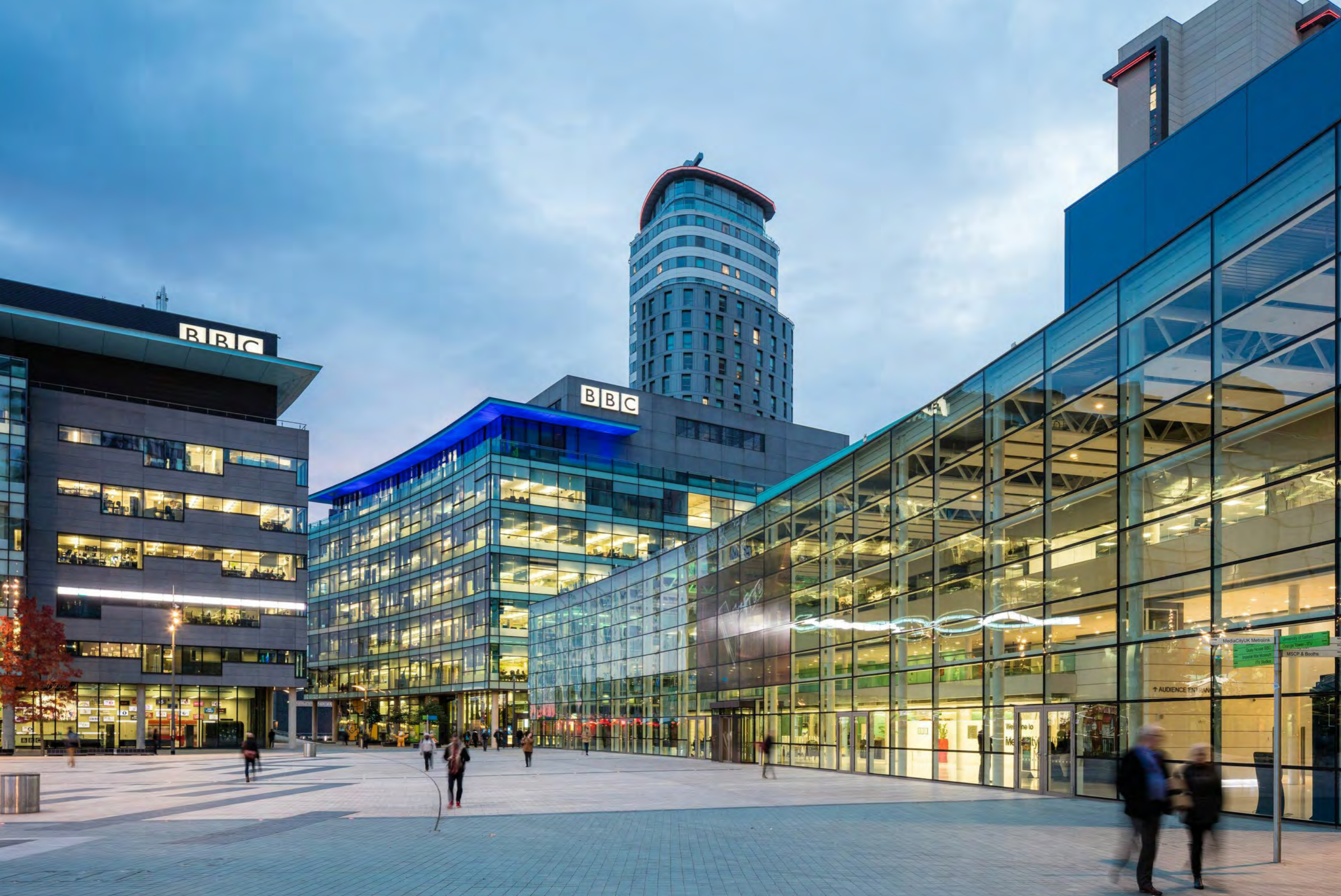
Fig.3.46 View of BBC buildings and Media Piazza
